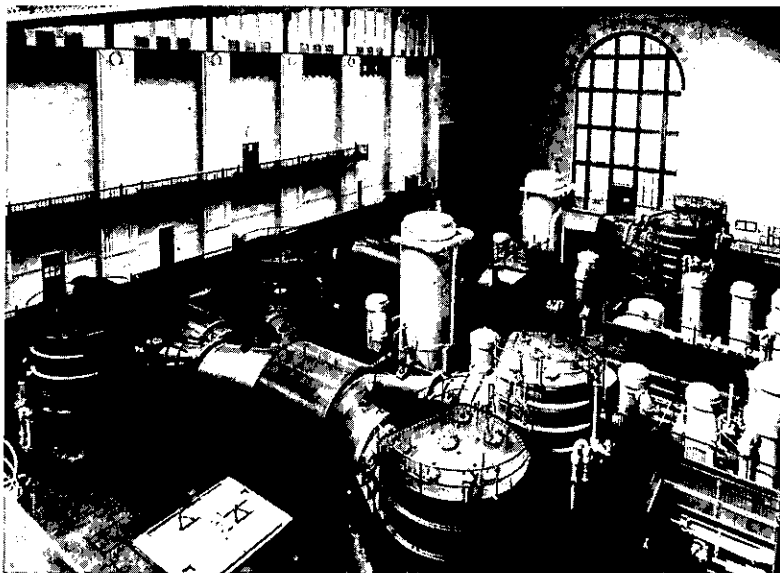
Three-unit, 208,000-kw turbine generator at State Line Power Station, Hammond, Indiana.
