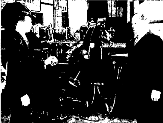
Television projector designed by E.F.W. Alexanderson and demonstrated at Schenectady's Proctor's Theatre.
