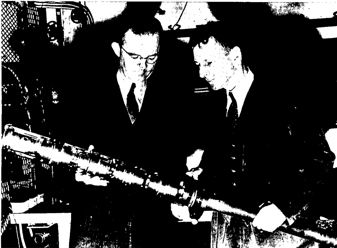
Ernest E. Charlton (l.) and William D. Coolidge with 900,000 volt X-ray tube.
