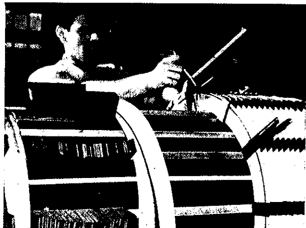
Winding transformer coil at Pittsfield Works.
