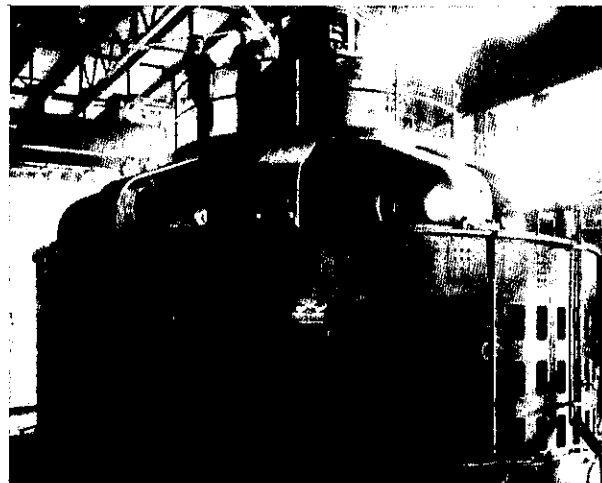
65,500-kva generator for the Niagara Falls Power Company.
