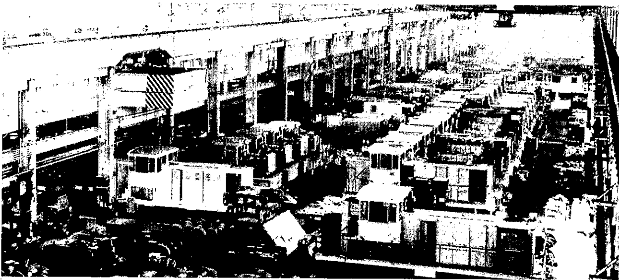
Diesel-electric power for military railroads — locomotives under construction at the Erie Works.
